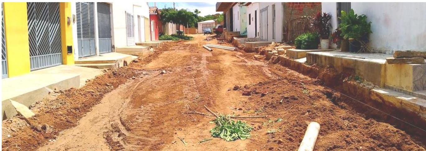
IMAGEM 02: TERRENO COM TERRAPLANAGEM EXECUTADA
